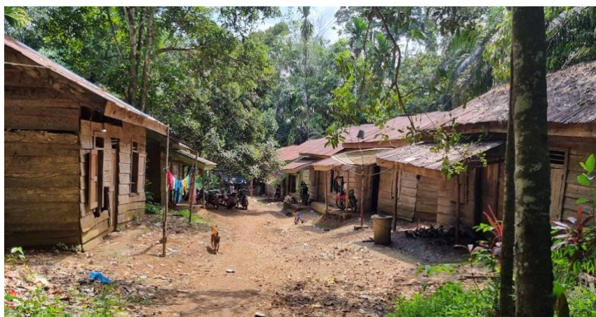
Figure 3. The condition of a SAD settlement in a village in Merangin Regency, originally established by the government. Many of the wooden structures are now damaged. The settlement is located on the edge of the village, near a public cemetery (Field Notes, 2024).
