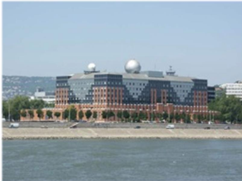
Northern building (room codes like: LÉ -1-22; LK -3-66)
